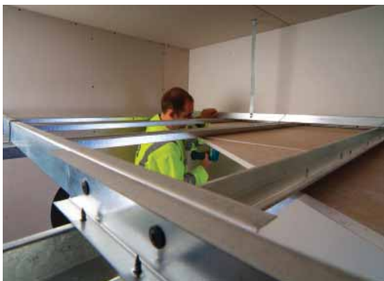
Speedline MF Suspended Ceiling System is ideal for commercial and domestic applications
